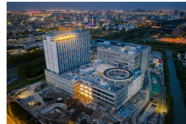
The research hospital under construction.
